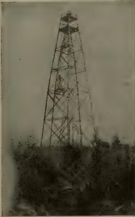
FIG. 16. Eighty-foot Tower. (Coast and Geodetic Survey.)
